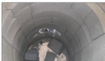
**Mitered:** Narrow, large pieces are more fragile and likely to damage in transport. The mitered pieces are stacked on a pallet, creating friction.
