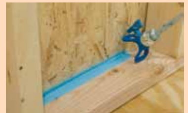
EcoSeal spray sealant should be sprayed on all joints, gaps and seams prior to insulation.
